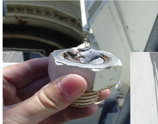
Case b, crack in bolt (FAT 50)
