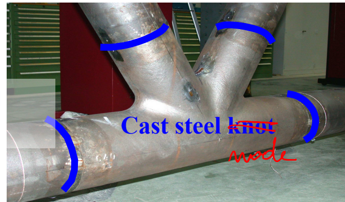
Conventional butt welds
